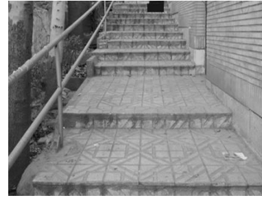
a. Before Rehabilitation
