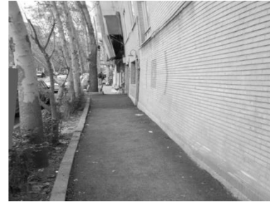
b. After Rehabilitation
