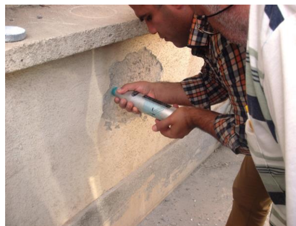
Figure 3: Schmidt hammers testing.
