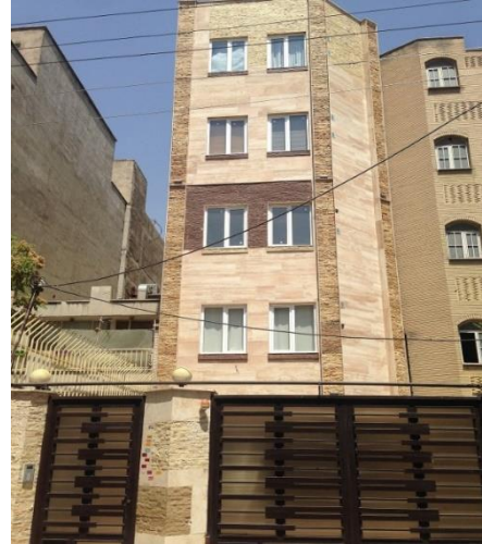
Fig. 4. 4-storey residential building located in Tehran – Iran
