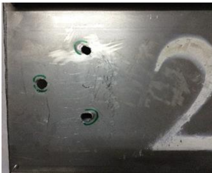
Fig. 8. Deformation mechanism of test specimen No. 2.
