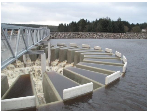
Fig. 2. Papaya spillway, Black Esk Dam, Scotland, UK [10].
