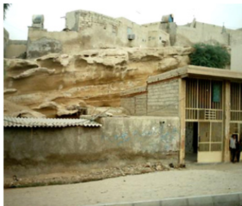
Fig. 4. Buildings with poor structures in hazardous place
