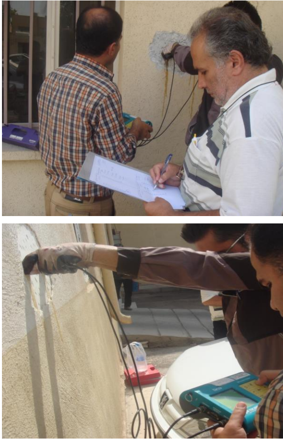
Figure 4: Ultrasonic testing in one side of the wall.
