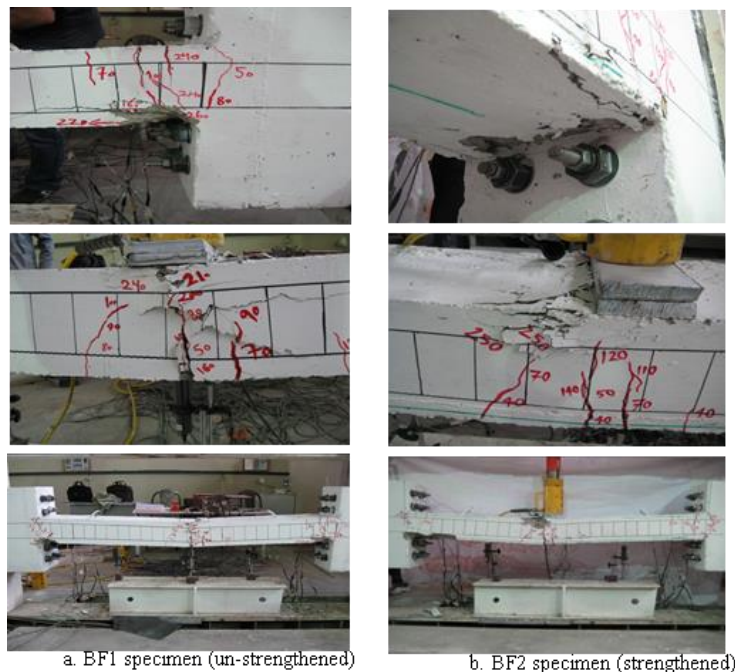
Fig. 5. Flexural failure in two fixed end specimen.
