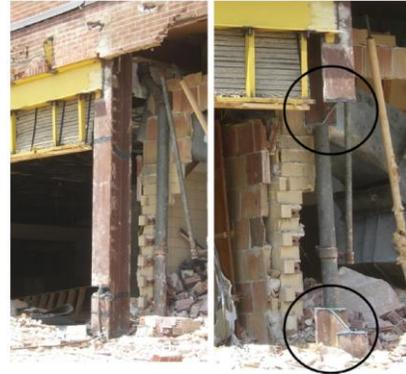
Fig. 6. Before and after removal of middle part of a column [14]
