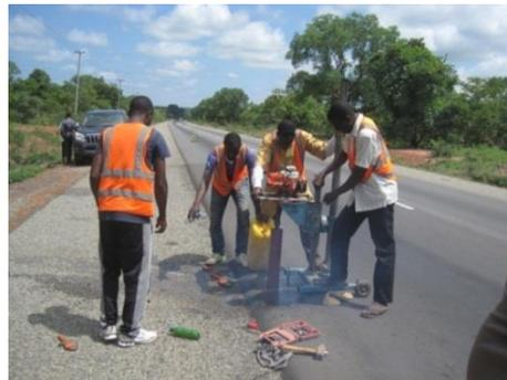
**Fig. 2.** Coring through the pavement structure..
