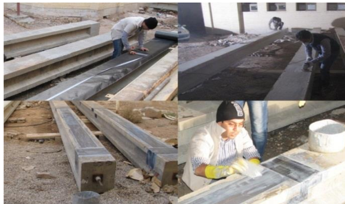
Fig. 3. Strengthening of UHSSCC beam
