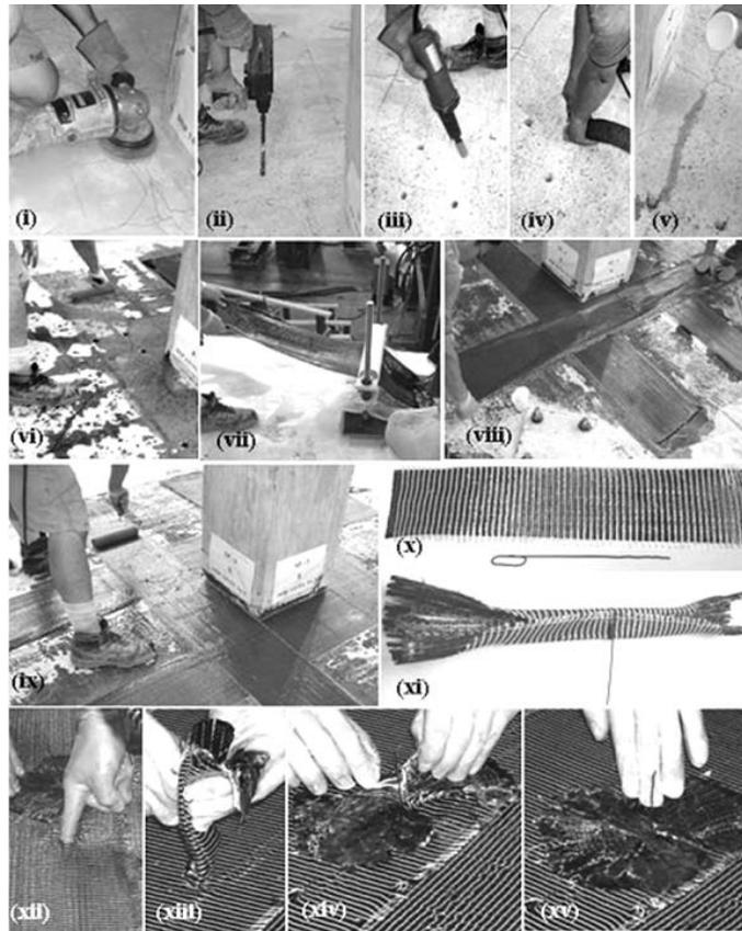
Fig. 7: Repair and strengthening process using FRP fan technique [11]
