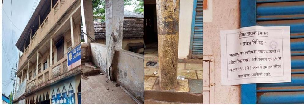
**Fig. 9.** shows the authorities' seal where the building is declared unfit to use under the C -3 category where entry of any person is not allowed (Dangerous building- entry restricted) written on the seal of the paper in Devanagari or Marathi script.
