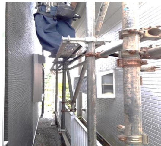
Fig. 2. Improper placement of support clamp (left) and corroded scaffold elements.
