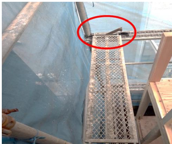
Fig. 2. Improper placement of support clamp (left) and corroded scaffold elements.
