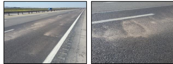
Fig. 8. Section 2 of 24 km, movement of mud from the lower layers to the upper layers after precipitation.
