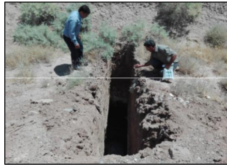
Fig. 15. Longitudinal drainage channel
