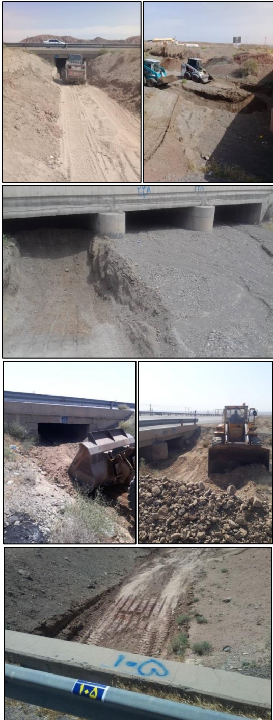
Fig. 14. Dredging bridges along the roadway to guide surface water.
