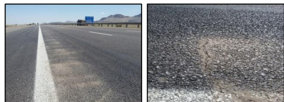
Fig. 10. Section 2 of 30 km, movement of mud from the lower layers to the upper layers after precipitation.
