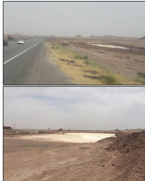
Fig. 16. Reinforcement of derivations and creating a water pit in the bottom line of the region to prevent flood entering and destruction of the Freeway.
