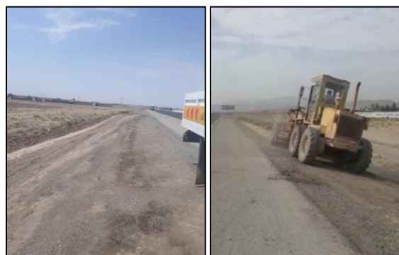
Fig. 13. Leveling shoulder and roadway and correcting the transverse and longitudinal slope
