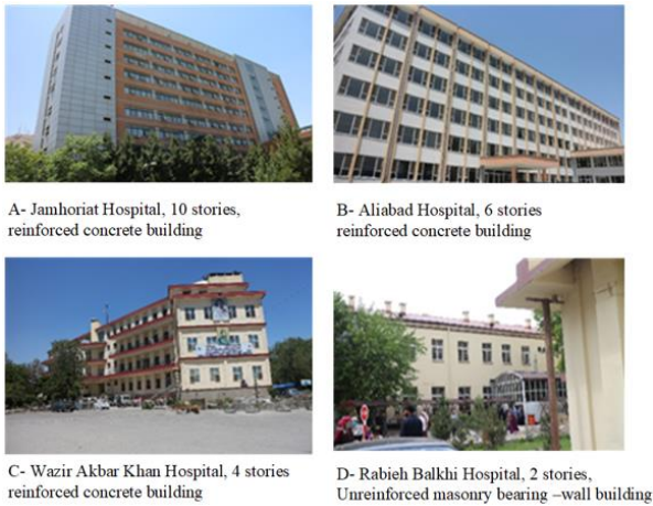
Fig. 3. Pictures of some hospital buildings in Kabul City.
