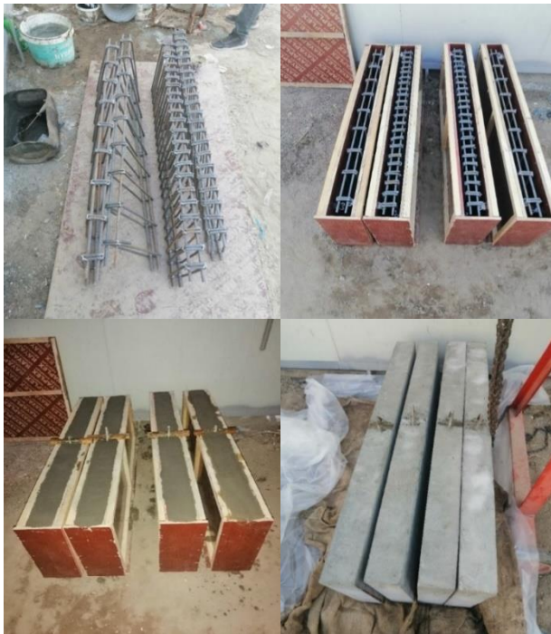
Fig. 3. Reinforcement, formwork, concreting of experimental specimens.
