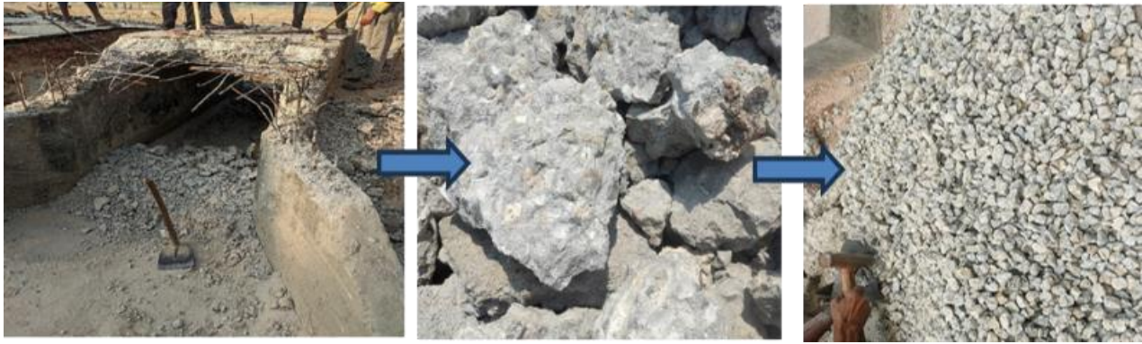
Fig. 1. Collection of parent concrete and making of recycled aggregate.
