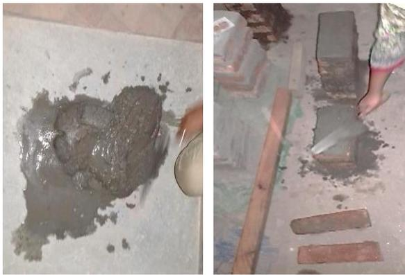
Fig. 13. Masonry Prism construction.
