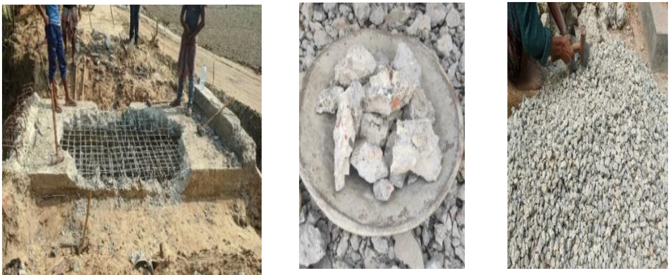
Fig. 1. Processing of recycled aggregate from demolished concrete.
