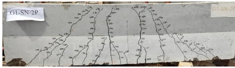
(a) Cracking map of the beam G1-SN-2P.
