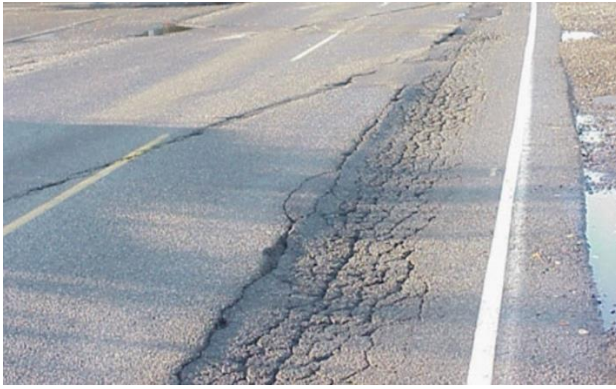
a) Cracks on pavement due to frost heaving
