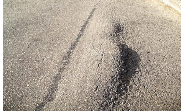
b) Upward bulge in pavement surface
