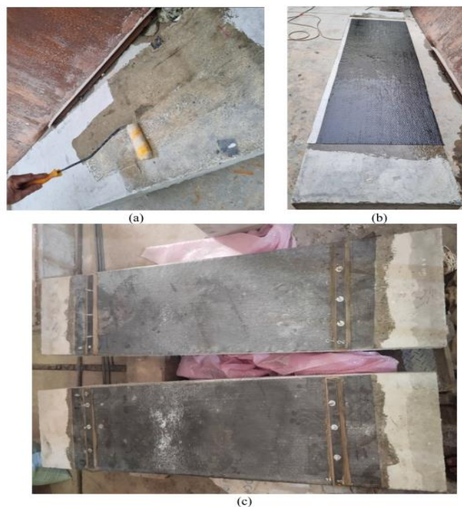
Fig. 33. Installing FRP layers with chemical anchors: (a) applying epoxy, (b) bonding CFRP to the concrete surface, and (c) placing threaded rods into concentric holes in steel plates and slabs.Adapted from Panuwat et al. (2024) [53].
