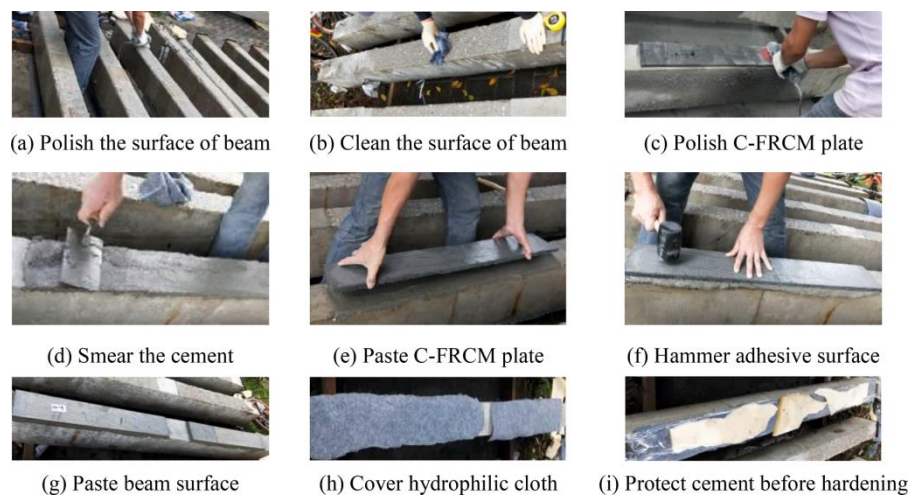
Fig. 8. Process of strengthening with prefabricated C-FRCM plate. Reproduced with permission from Feng et al. (2022)[23].
